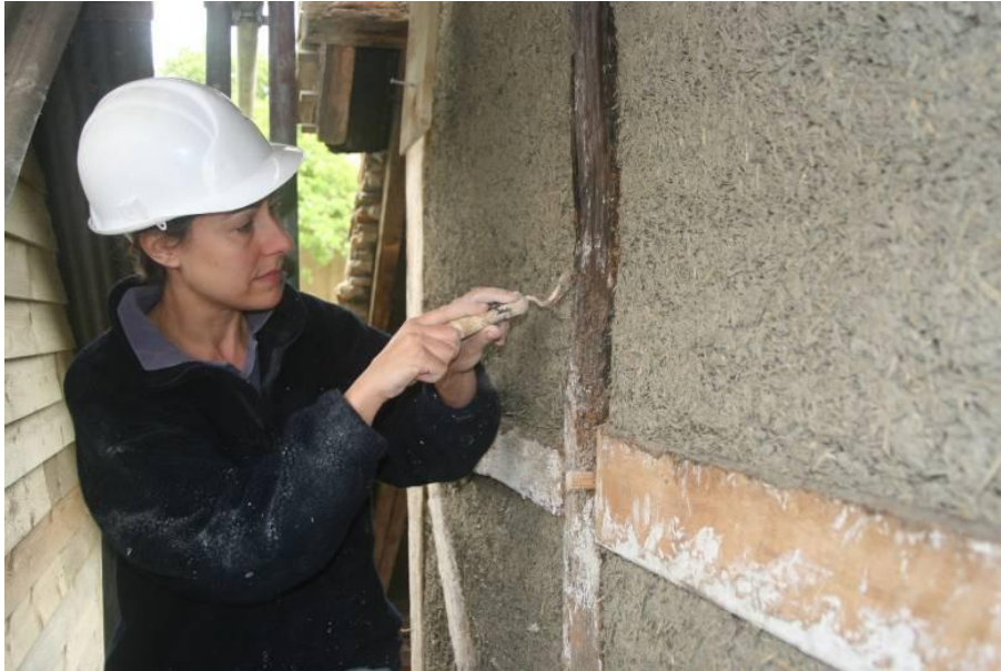
Fig. 27 Hempcrete infill in timberframe (source: www.limetechnology.co.uk)
