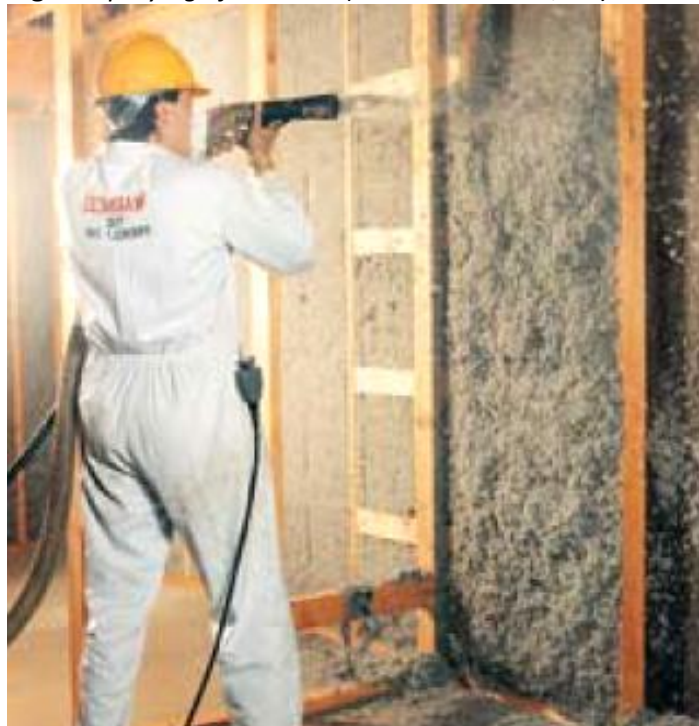
Fig. 33 Spraying of cellulose (source: Warmcel, UK)
