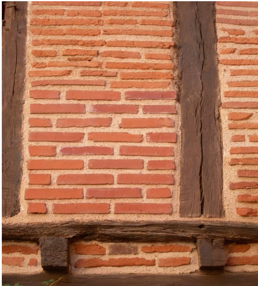
Fig. 21 Renovation in Albi with old and new bricks (H.Valkhoff)
