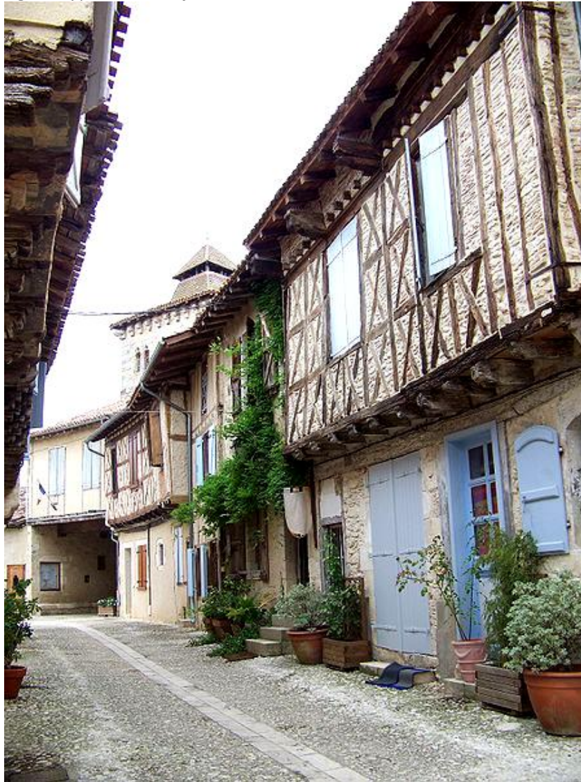
Fig. 36 Typical timber-frame street in SW France, in Sarrant (Wikipedia)
