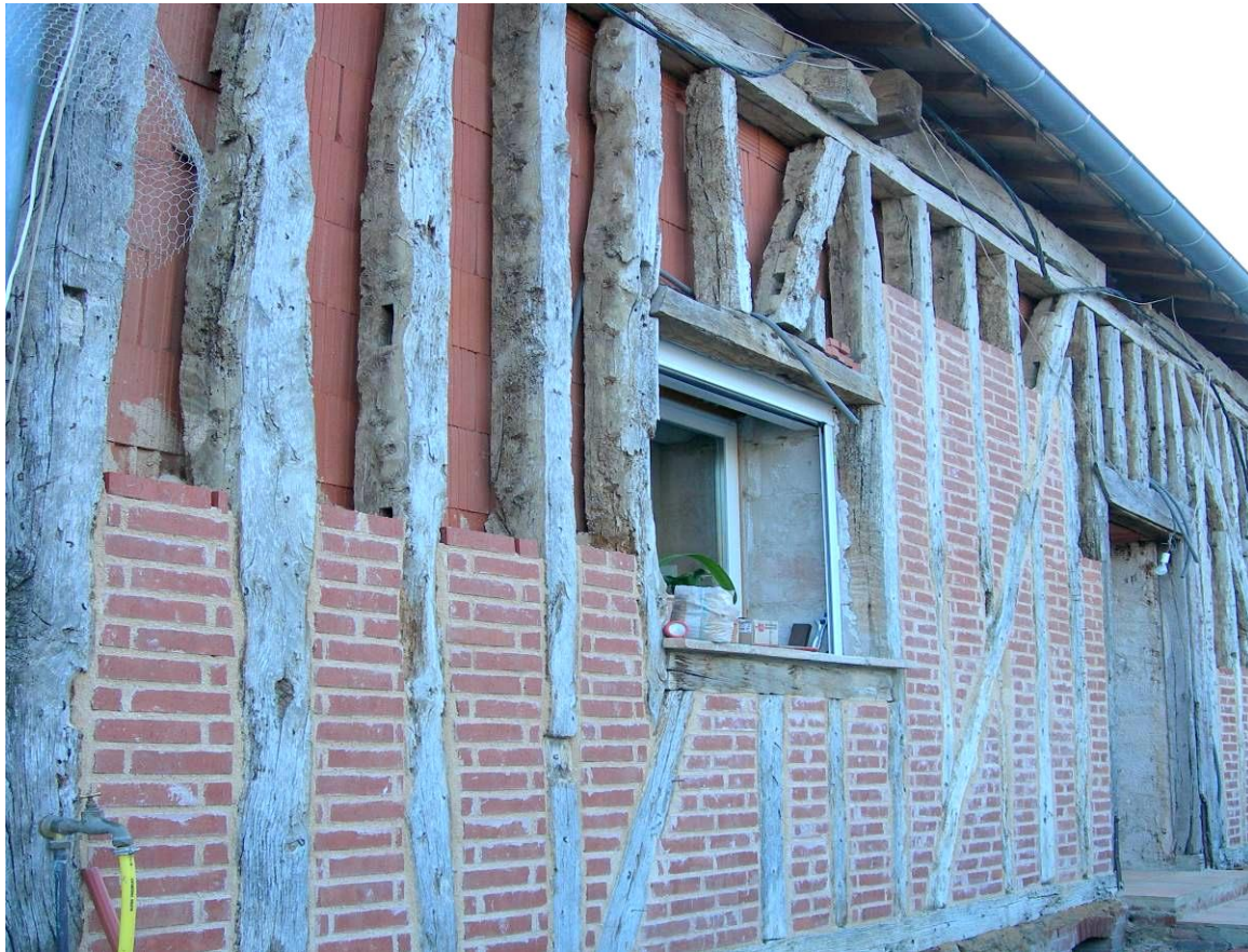
Fig. 11 Timber-frame with brick infill and monomur insulation (H.Valkhoff)
