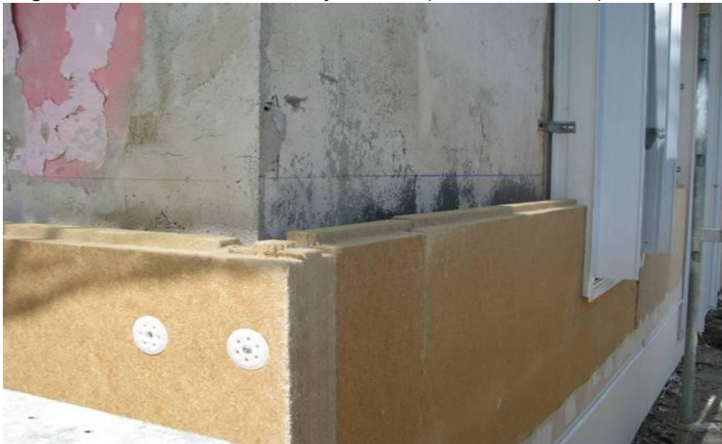
Fig. 25 Exterior insulation with woodfibre board (Floissac et al., 2008)
