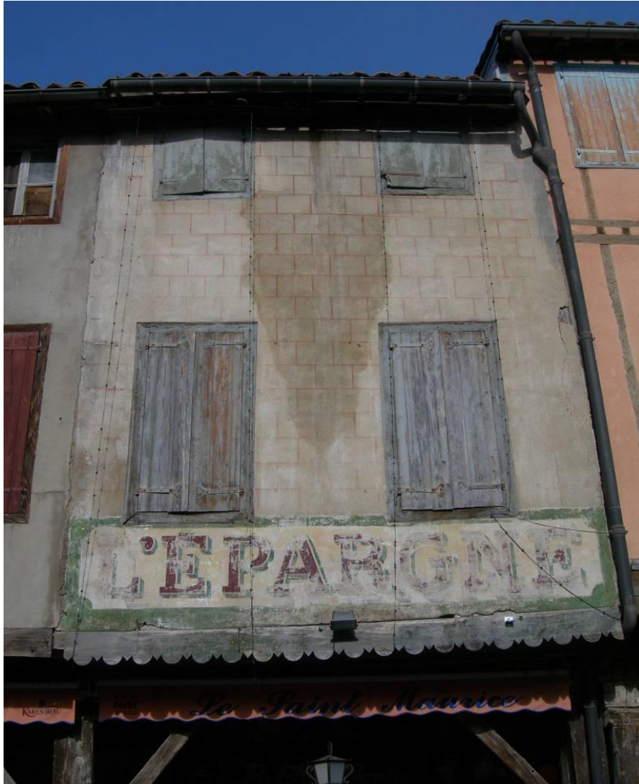
Fig.38 Old renovation made timber-frame house look like stone (H.Valkhoff)
