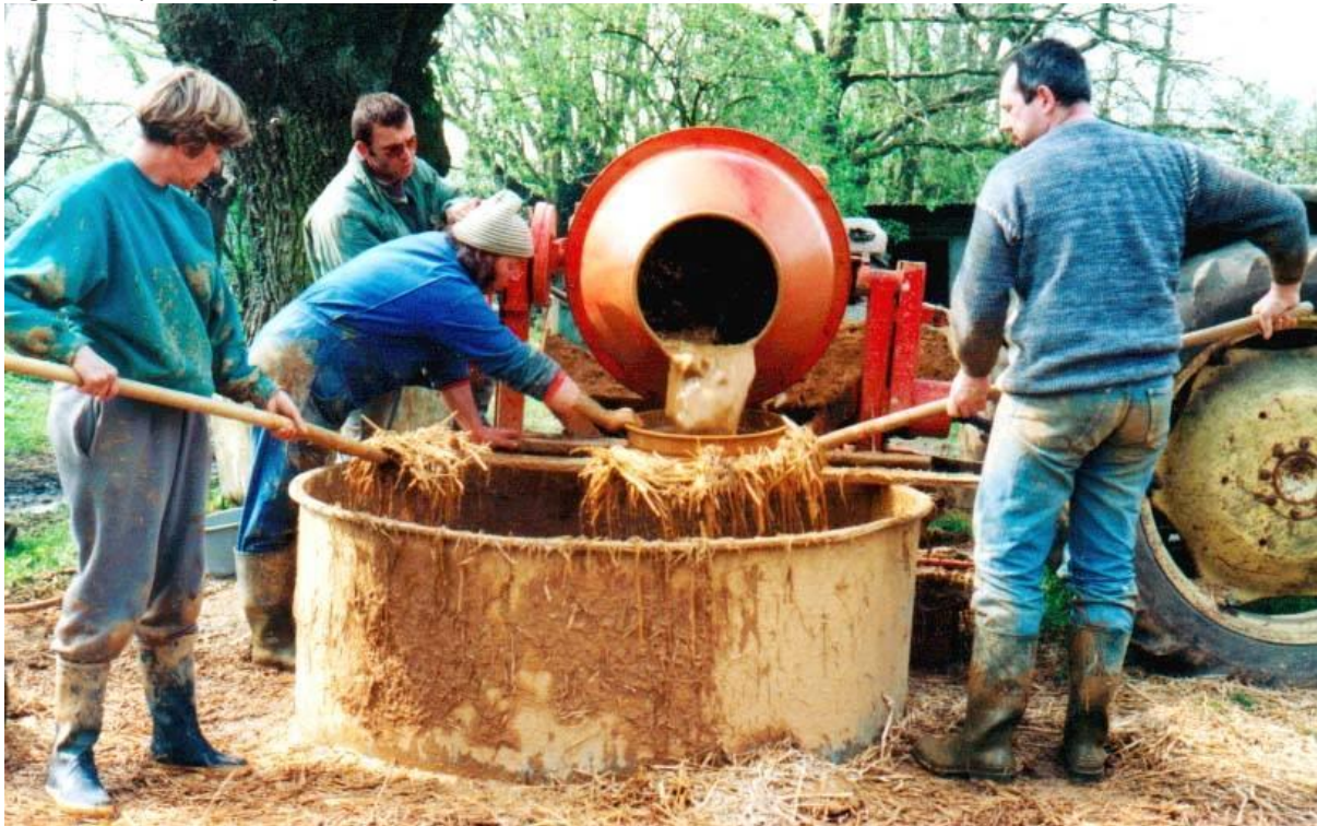
Fig. 26 Preparation of earth&straw mix in SW France (Marcom, 2002)
