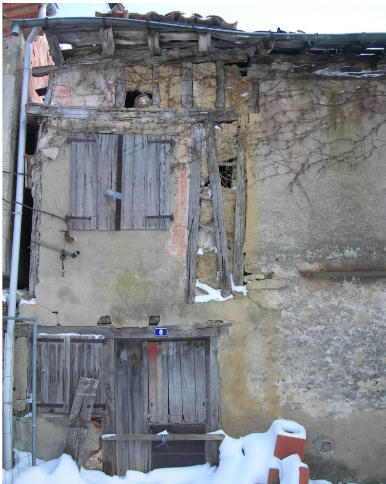
Timber frame house with wattle& daub in ruins (H.Valkhoff)
