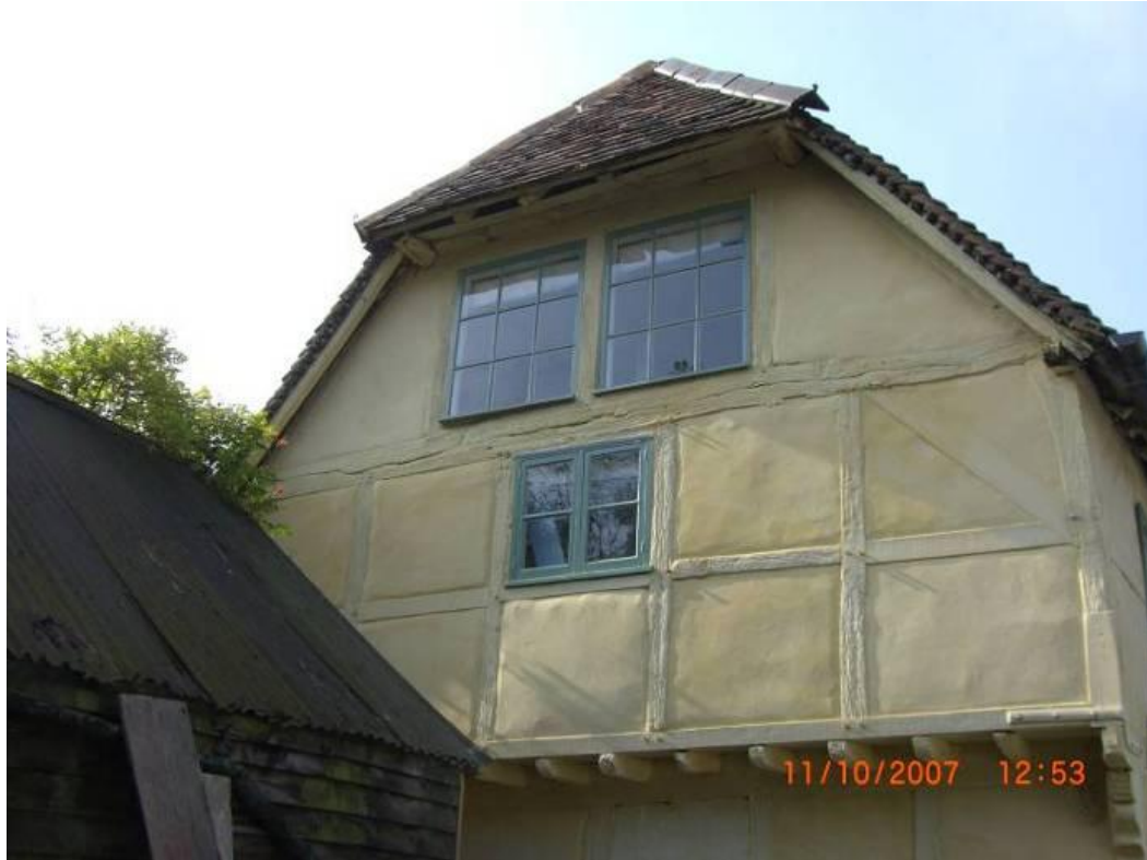
Fig. 37 Timber-frame house with hempcrete infill in the UK ( www.limetechology.co.uk )
