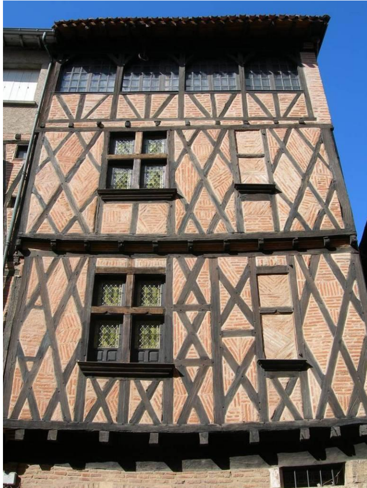
Fig. 1 Typical timber-frame with brick infill in Albi (H.Valkhoff)
