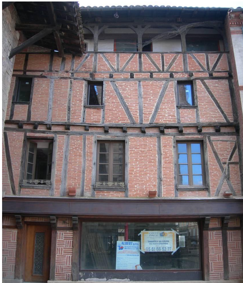
Fig. 23 Renovation of timber-frame building in Albi (H.Valkhoff)
