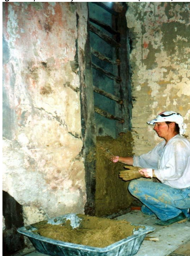
Fig. 35 Reparation of wattle and daub (Marcom, 2002)
