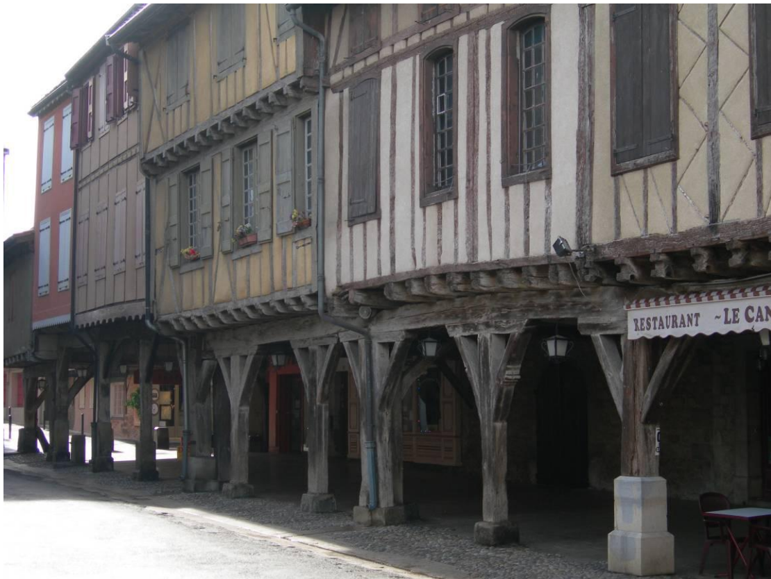
Fig. 5 Timber-frame with render onto daub in Mirepoix (H.Valkhoff)
