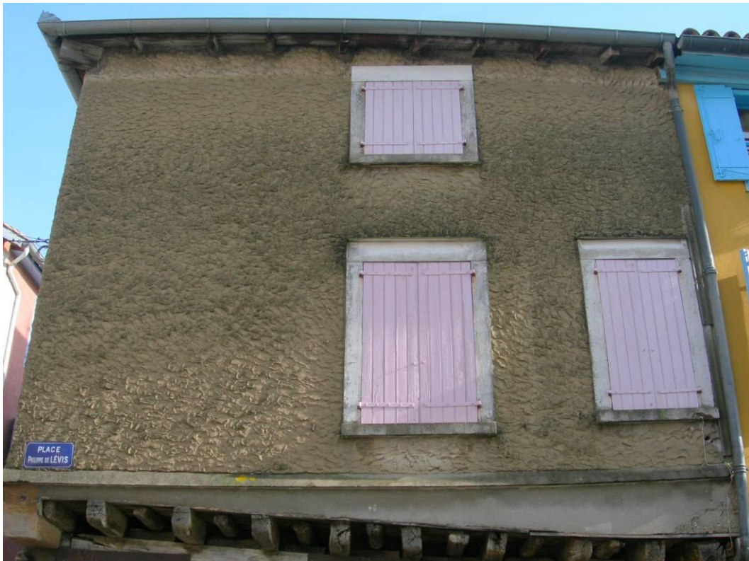
Fig. 22 Example of cement render onto period timber-frame in Mirepoix (H.Valkhoff)
