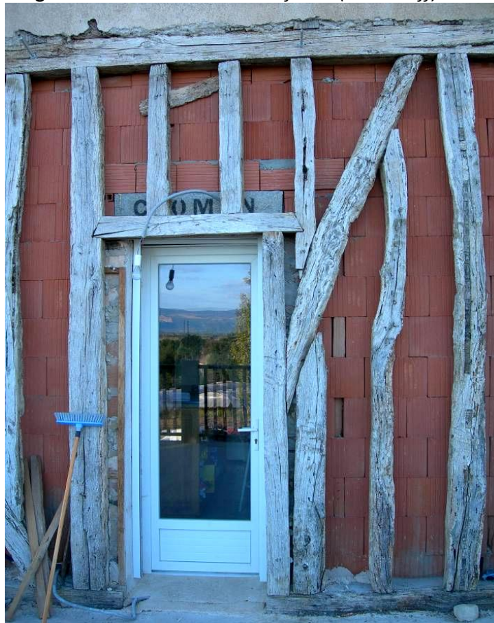
Fig. 29 Monomur behind timber-frame (H.Valkhoff)
