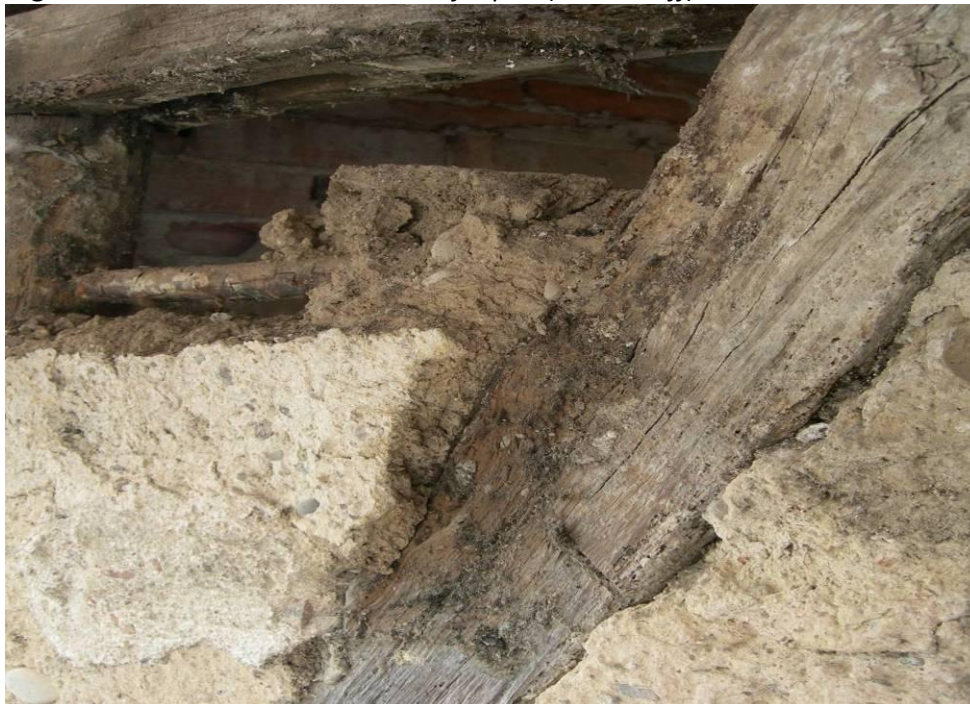
Fig. 34 Old wattle and daub in need of repair ( H.Valkhoff)
