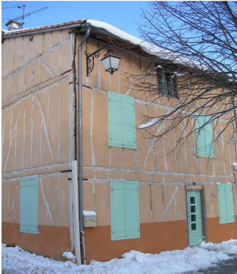
Fig. 2 Renovated timber-frame house in Puylaurens (H.Valkhoff)
